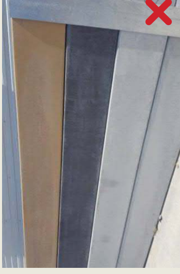
Figure 5 - Concrete Sleeper Retaining Wall
