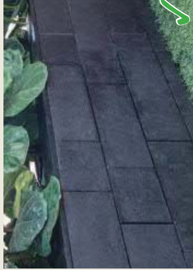
Figure 4 - Charcoal coloured smooth faced masonry block
