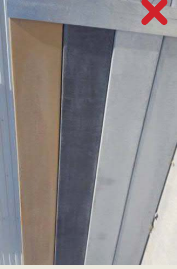
Figure 5 - Concrete Sleeper Retaining Wall
