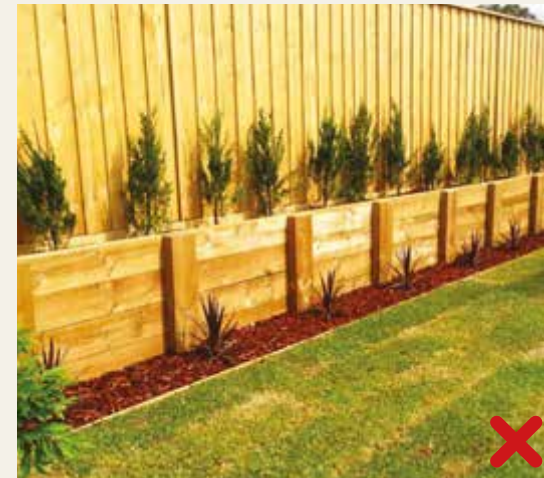
Figure 6 - Treated Pine Retaining Wall
